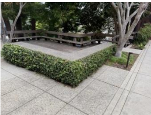
Existing back side of the courtyard wall that would remain unchanged
